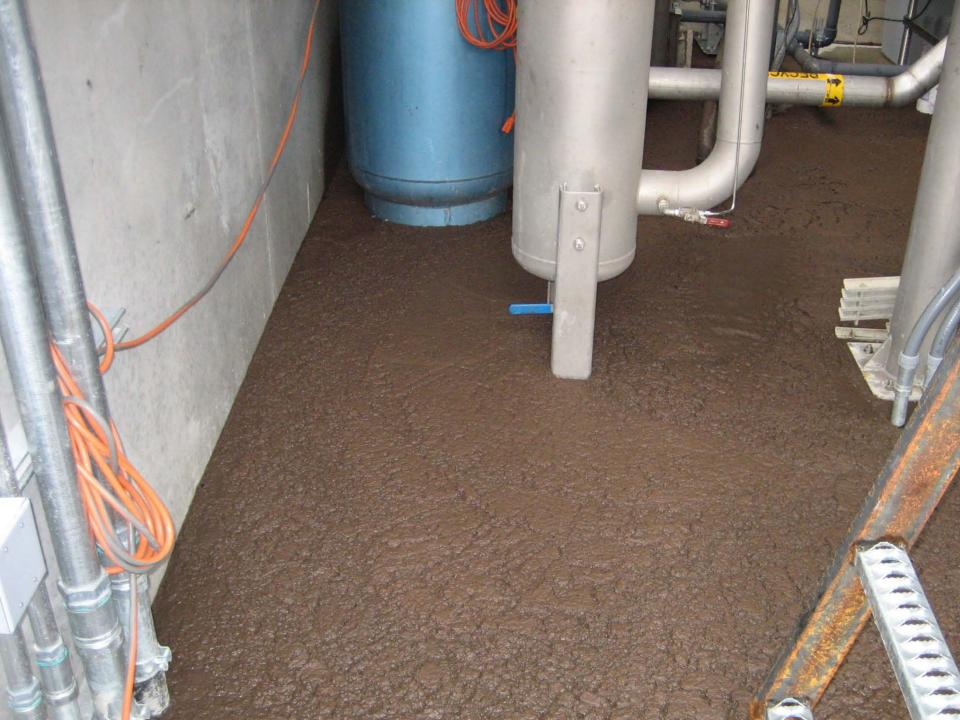
Never put your waste water sludge into a big. plastic tank for storage without any aeration or the sludge will immediately go septic, discharging dangerous levels of hazardous hydrogen sulfide gas and other noxious odors that are not conducive to pleasant dining in a nearby beer garden or healthy operation of a sludge press.
