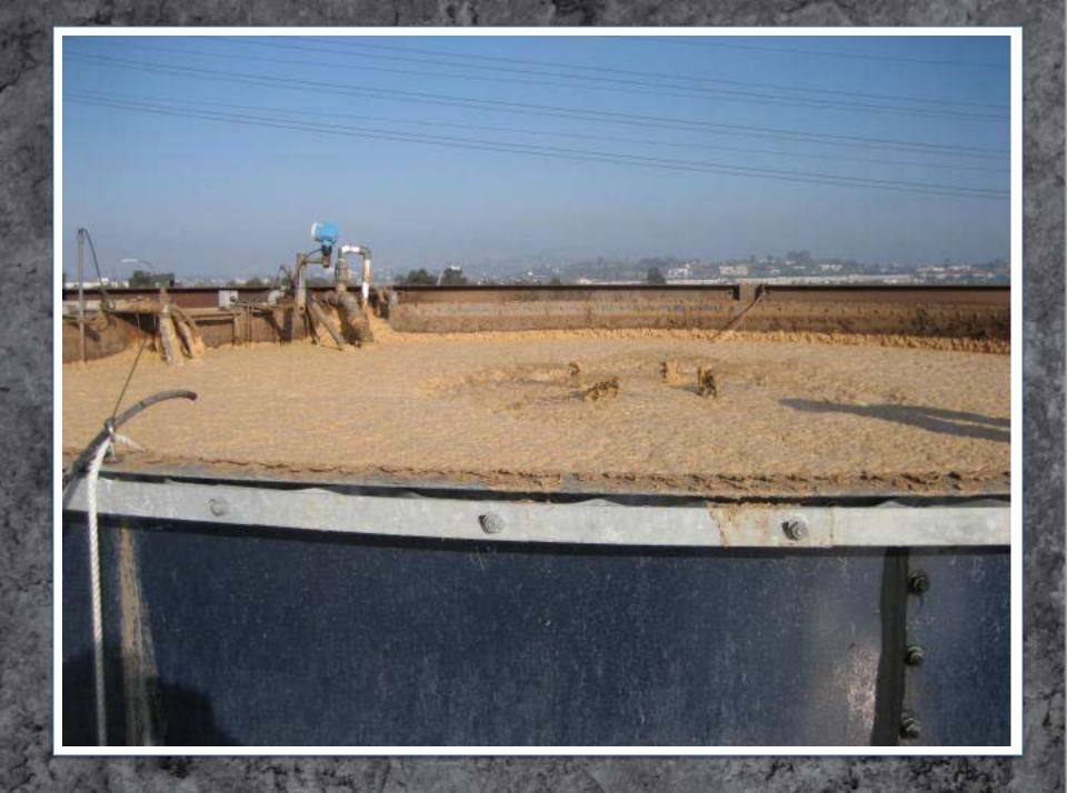
Never pump your waste water and return activated sludge into the top of your aeration tank and then draw off your effluent for separation from the top of the same tank. You will wind up processing the same sludge over and over and the high strength BOD will take a shortcut from inlet to outlet, the bugs will not get fed and the BOD of the final effluent will often be out of range of the permit limits.
