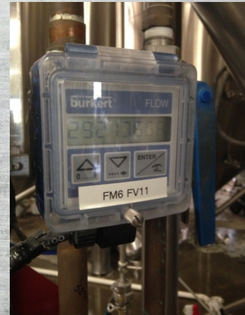
Flow Meter w/ 4-20 output
