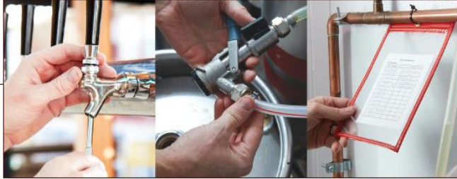
Figure 7.29. Faucets and couplers should be inspected visually to ensure that proper line-cleaning frequency and procedures is being followed. Straws can be used to look for soil inside faucets. Line cleaning logs should be maintained.
